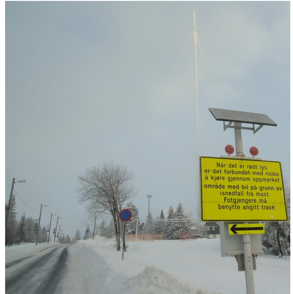
Warning system at Tryvann communication mast, Oslo, 2015.
